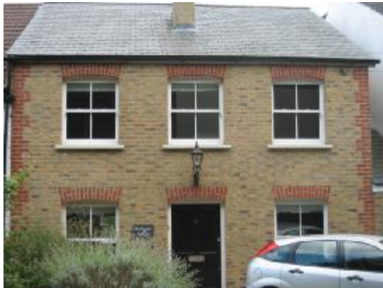
Willingale Cottage, No. 21, building of townscape merit
