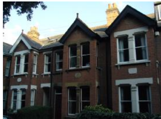
The Four Sisters, 35-45 Staples Road, building of key townscape merit
