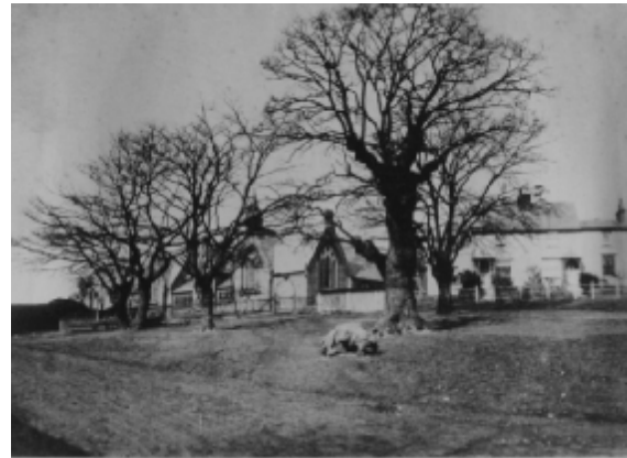
View of the Original School c1890
