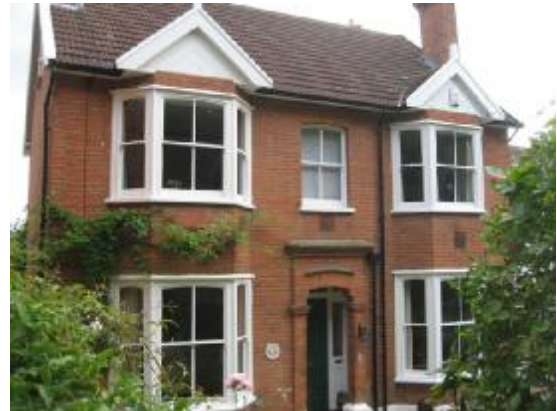
Forest Lodge, No. 5, building of townscape merit
