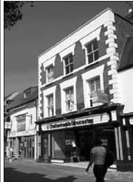
One of the buildings in Waltham Abbey on the 'Local List'.
