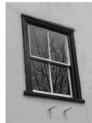
Satisfactorily repaired sash window.
