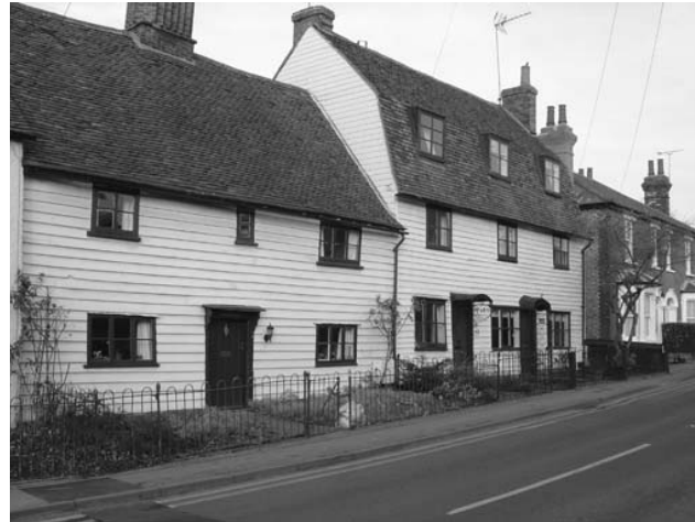
The Niche, St Anne's Cottage & Dowsett's House, Harlow Road, Roydon
