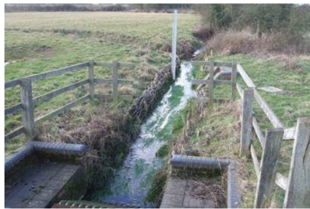
Drainage ditch looking west from culvert
