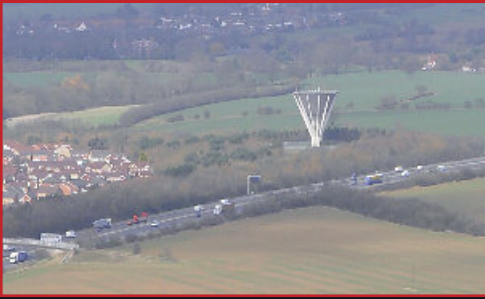
Church Langley Water Tower is on the edge of the Stansted CTR
