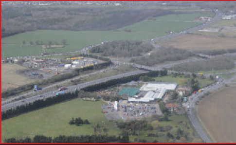
The M11 Junction 7 roundabout at Harlow – 20 base leg turning point
