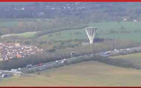
Church Langley Water Tower is on the edge of the Stansted CTR
