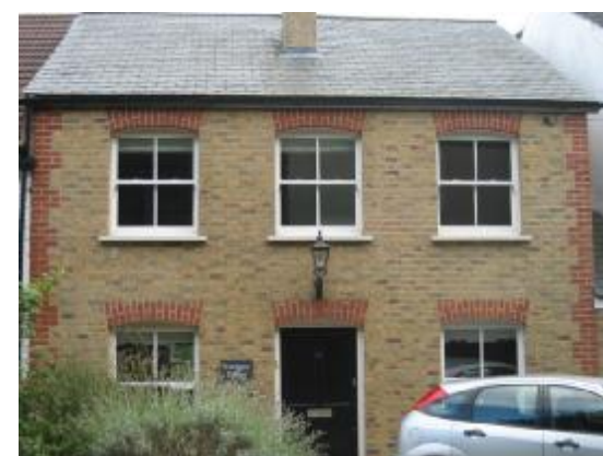
Willingale Cottage, no. 21, building of townscape merit
