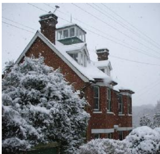
Forest Villa, no.7 Staples Road, Locally Listed
