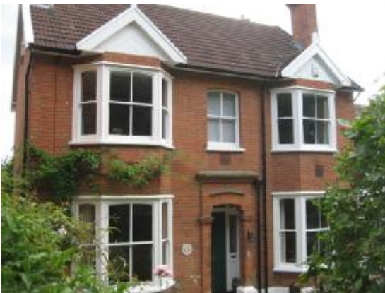
Forest Lodge, no. 5, building of townscape merit
