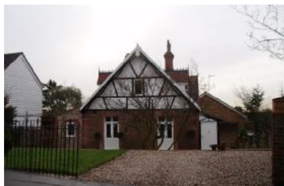
No.3 Melbourne Cottage, Locally Listed
