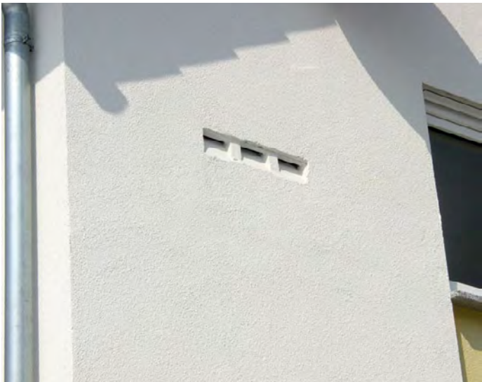
Bat tubes (3no.) integrated within a rendered finish (ref: Schwegler Natur)
