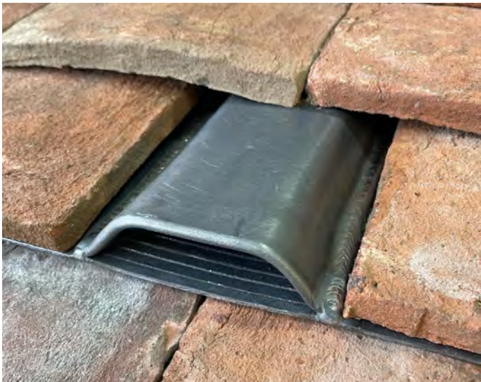
Bat tube for slated & tiled pitched roofs (ref: Just Lead)
