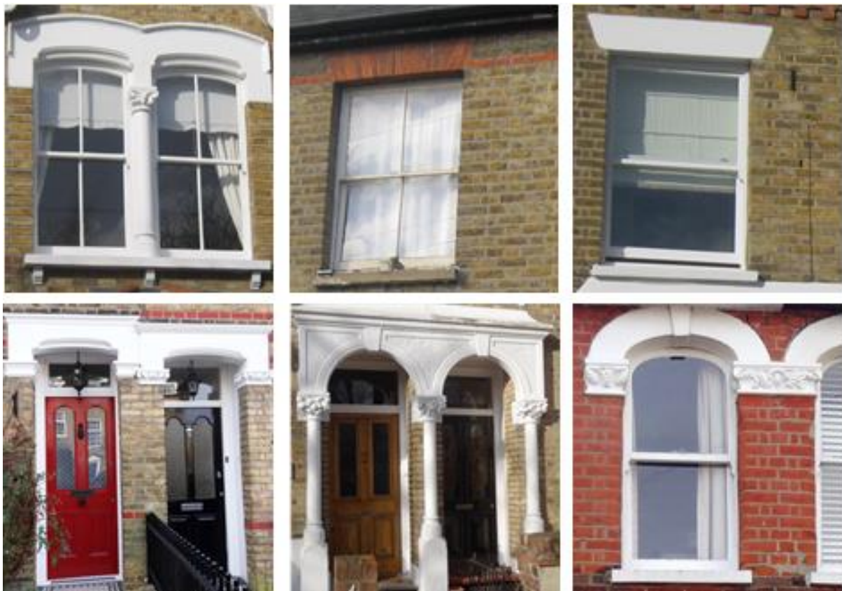
Figure 36: Timber windows and doors (historic and replacements)
