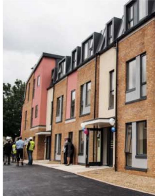
Homes for Heroes self build scheme in Bedminster Bristol with The Community Self Build Agency (CSBA) and Knightstone Housing Association http://www.self-build.co.uk/homes-heroes
