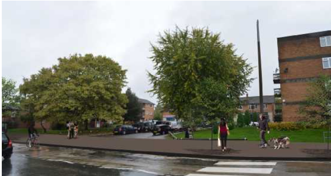
Improved Pavements & Crossings
