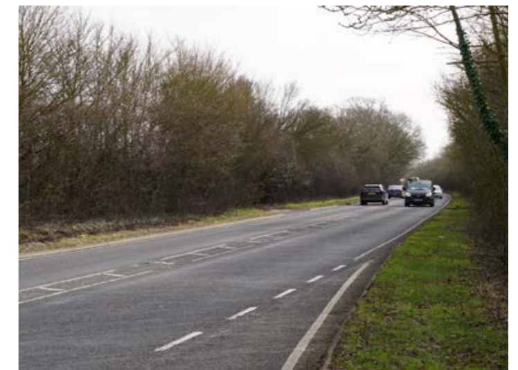
Looking east along A414 from junction with Vicarage Lane West (view 5)
